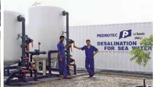
Design, Construction, Installation and Commissioning of: Sea Water Electrochlorination Plant. 2x22 Kgs/ h Pure Chlorine Production.
